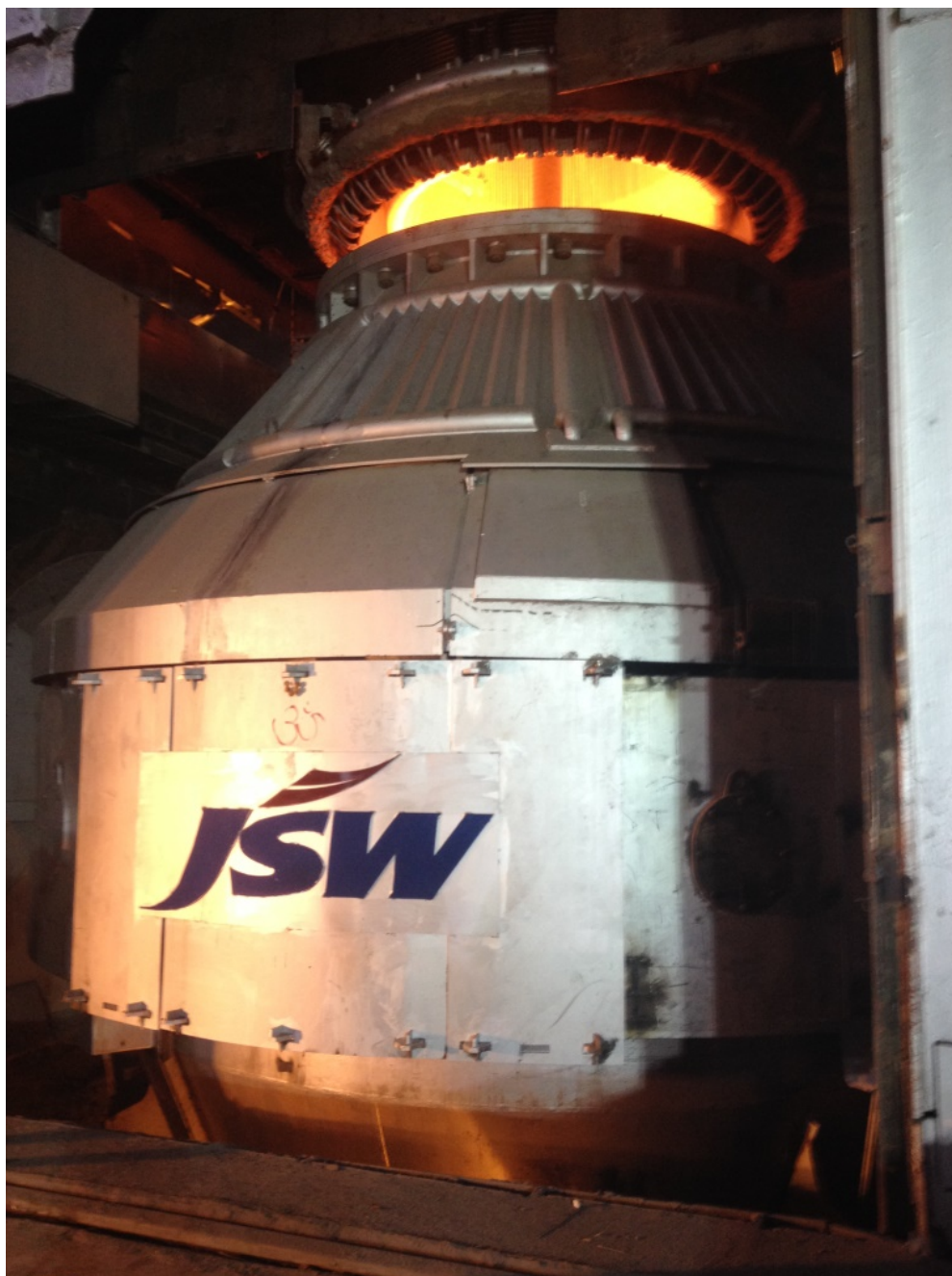
LD (BOF) converter from Primetals Technologies in the Steel Melt Shop no. 2 in Vijayanagar, Toranagallu, India of JSW Steel.
